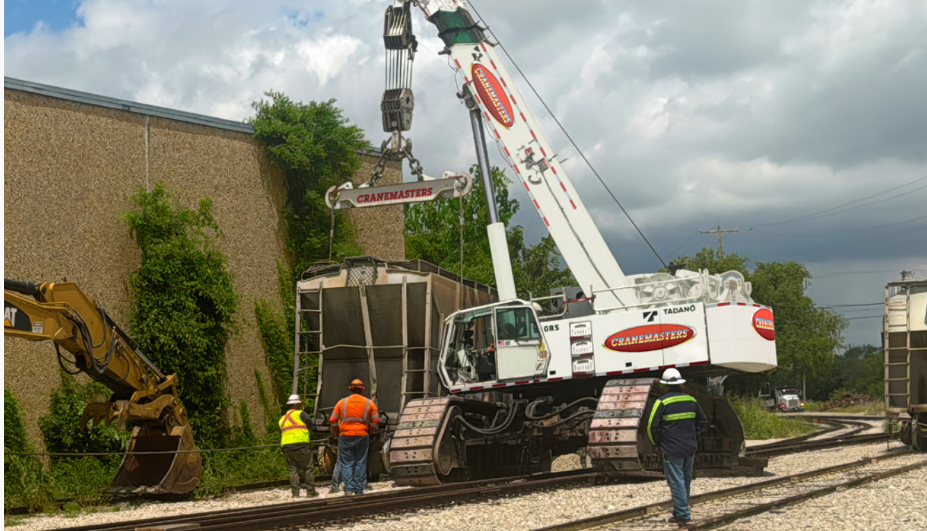
The 1-Side • 1-End™ approach in action as Cranemasters rerails a car just a few feet from a warehouse building.
