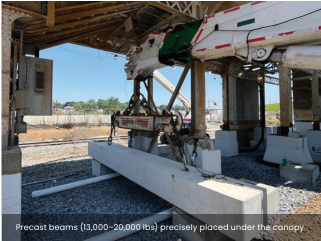
Precast concrete panels (11,000–32,000 lbs) lifted from semi trailers and positioned under the canopy.
