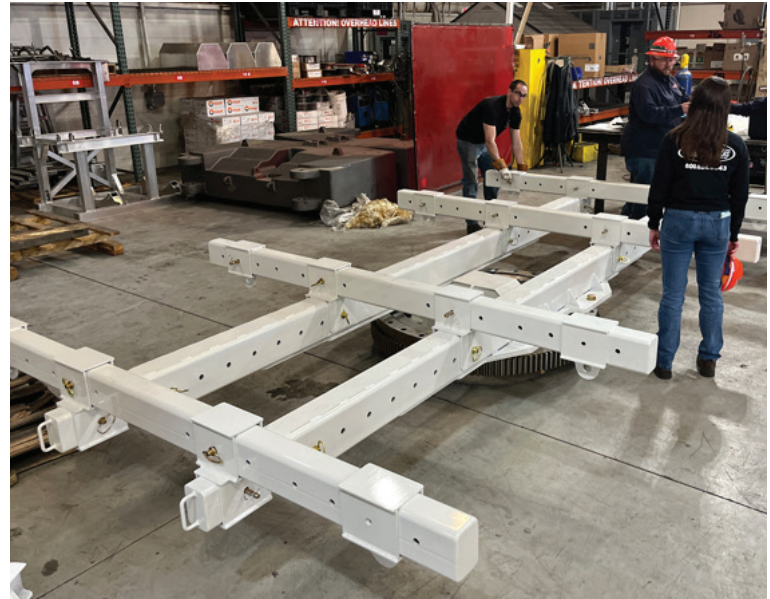
Building the custom lift beam
