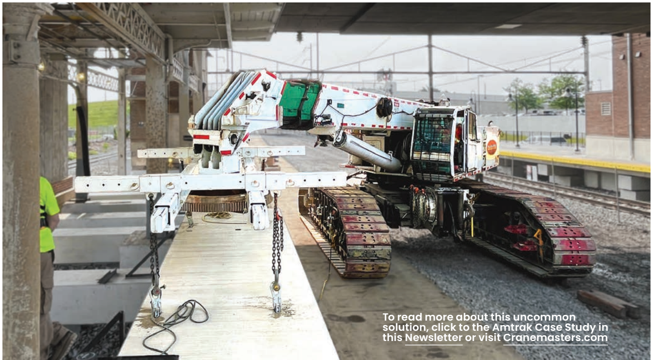
The Cranemasters 200 RS Crawler placing a large precast concrete panel utilizing the purpose-built lift beam
