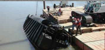
Transition from land to water is very possible with our equipment. By loading cranes on spud barges, we are able to retrieve train cars and equipment from lakes, rivers and creeks.
